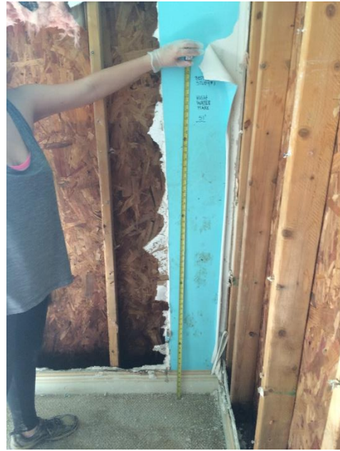
Figure 3 - Leave one vertical section that includes the wall material and base board as well as special conditions (built-in shelves) . Step back and take a photo showing the wall and tape measure. Use high resolution photographs.
